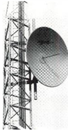
Fig. 20. Solid parabolic STL antenna. This type of antenna provides excellent side and back lobe protection and is used in situations involving channel sharing. (Courtesy Andrew Corporation)
