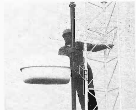
Fig. 24. Radome used on single bay FM antenna.
