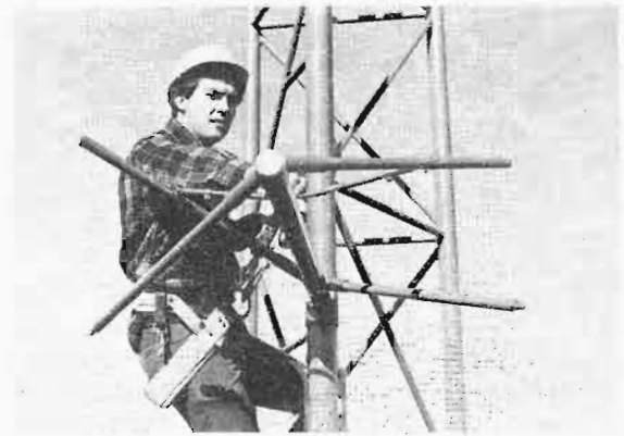
Fig. 23A. Rigger installing Cpol radiator to lower leg.
