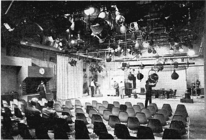
FIG. 3-3a. WRGB-TV. Showing counterweighted pipe batten in lowered position.
