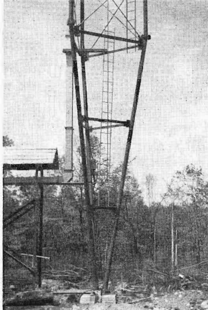
FIG. 2-6. Photograph showing tapered-base-type tower.
