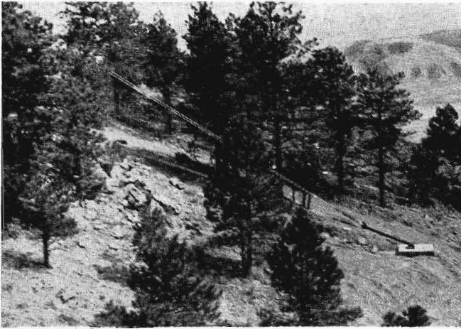
FIG. 2-63. Guy anchor installation at KOA-TV, Denver, Colo.
