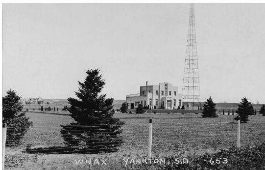
In 1936 WNAX built this modern two-story showplace transmitter building and tower five miles east of Yankton, which is still used by WNAX today.
