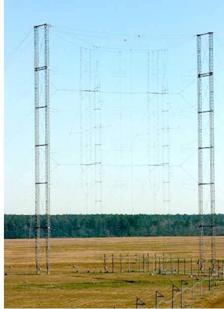
One of 19 curtain antennas roughly 300 feet high
