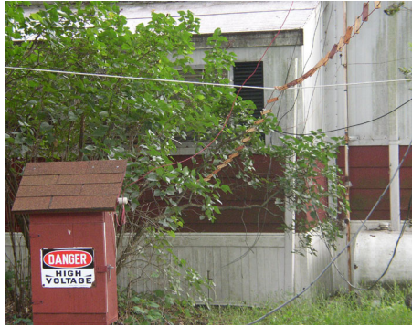
From the shack window, the feedline passes an antenna tuner "doghouse" ...
