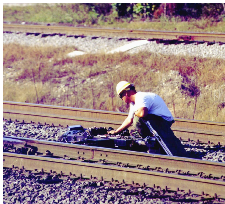
... a Norfolk Southern signal maintainer is working on a balky switch machine motor on one of the cross-over switches.
