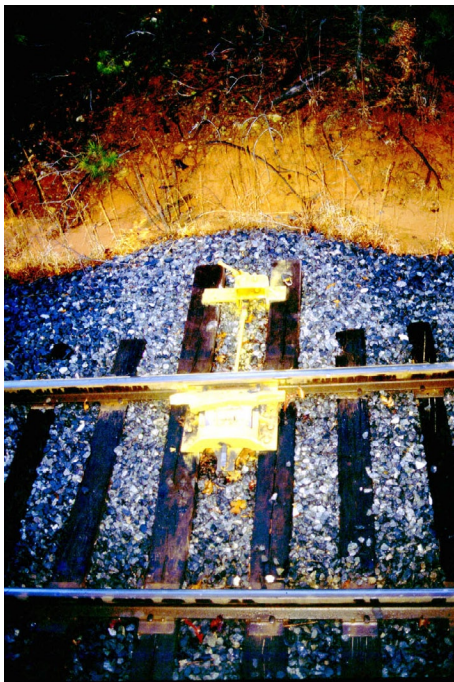
A permanently installed derail on an industrial spur has been moved to its off position allowing the industry's tracks to be switched. The photo was made from the cab of one of the engines that was still on the main line at that point.
