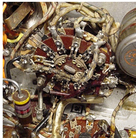
The base of the problem i.f. transformer (long screw protruding from center) can be seen between my large 5-watt replacement resistor and the back wafer of the “avc-off-mvc” switch.
