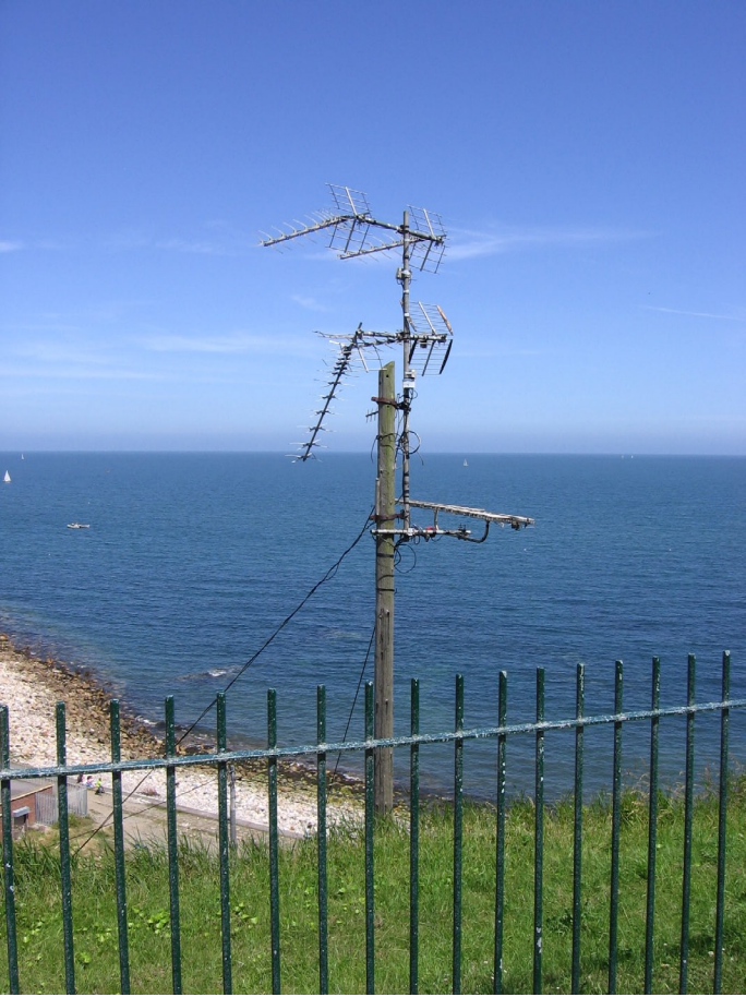
Antennae used by the museum's amateur radio station E10MAR. The station operates primarily on Sundays using Morse code on HF with 25 watts through home made 40 and 17 meter dipoles, as well as 2 meter FM. More info from the web site given at the end of the article.
