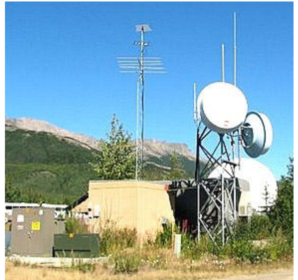
The Alaska Railroad communications complex at the train station.
