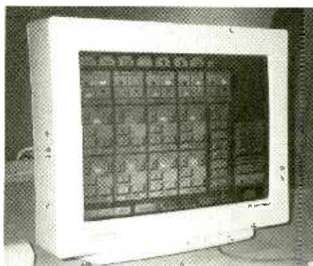
17" touch screen radio control/monitor screen which displays eight transmit/receive modules and 20 monitor modules. No more buttons! (Mouse/trackball also used to control functions.)
