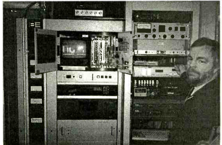
Bill Seier, WB0SIP, Chief Engineer, alongside the KFGE transmitter.
