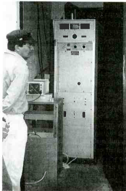
Radio Interoceánica's shortwave transmitter is a rebuilt RCA medium wave transmitter with 1,000 watts.
