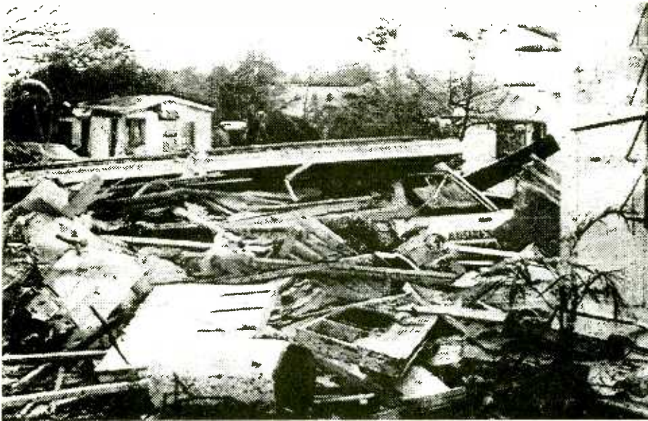
Housing is often severely damaged following a disaster. Enormous amounts of food supplies and plastic sheeting are ordered through the MATTS radio communication system.
