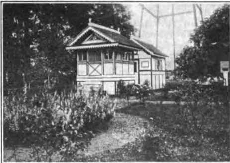
STATION BUILDING, POWER HOUSE AND BASE OF TOWER
