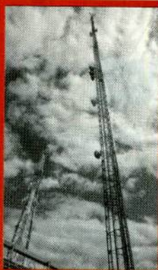
New tower construction has been tough going in several markets.
