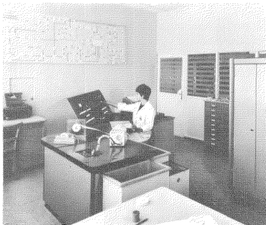
Figure 14—Stantec 2000 warehouse stock control and handling system.
