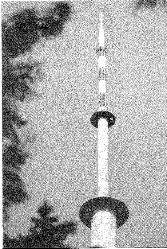
Figure 5—Antennas for television transmission on bands III and V.
