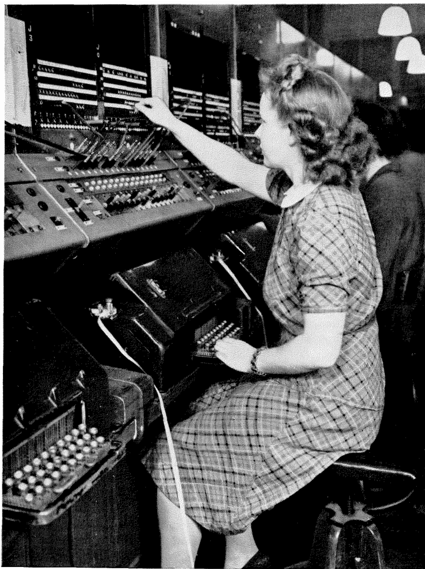
Manual teleprinter switchroom at Manchester, England.
