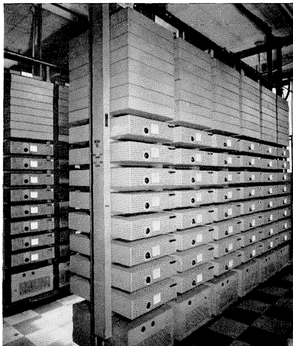
Voice-frequency carrier telegraph installation in a modern Western Union Telegraph Company office. Each vertical rack of carrier equipment (left) mounts 8 channels. The test board is at the right.
