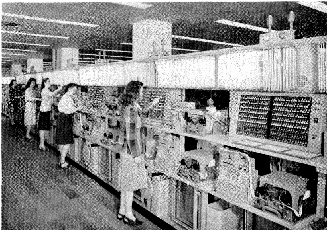
Push-button switching aisle in Philadelphia, Pennsylvania, office of Western Union Telegraph Company.
