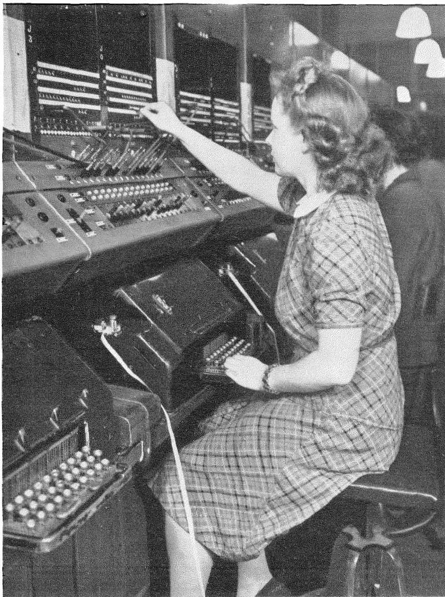
Teleprinter switch-room in Manchester.
