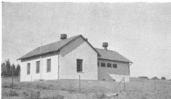
Fig. 13—Typical repeater station building.
