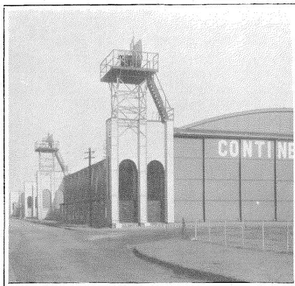
Fig. 4—View of the reflector towers at Lympne, England, terminus of the Anglo-French micro-ray link between Lympne and St. Inglevert, France. It represents the first commercial micro-ray installation, designed to operate on a 17-centimeter wavelength with sharply concentrated beams.
