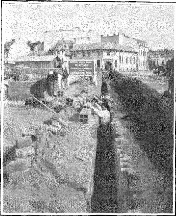
Placing Clay Conduit in Bucharest.
