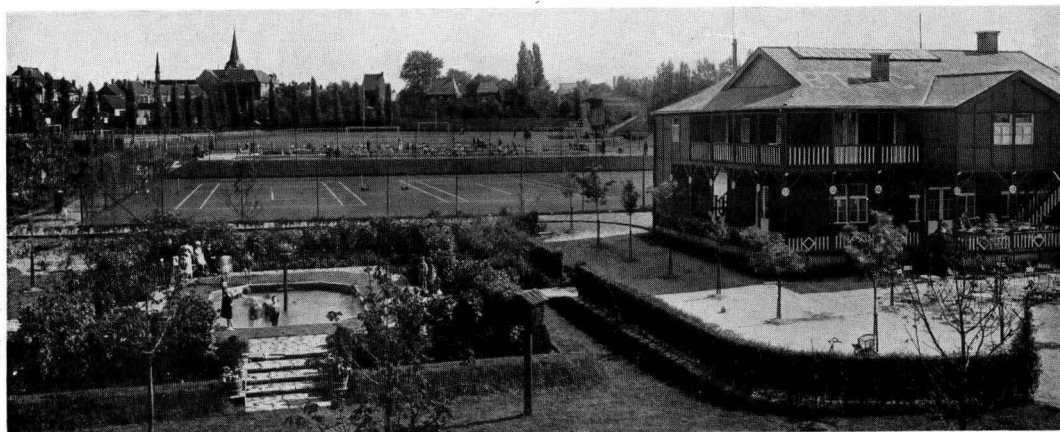
The sports and recreation grounds of the Bell Telephone Manufacturing Company, Antwerp, cover nearly 10 acres. They include a roomy club house, a playground for children with a children's swimming pool (visible in left foreground), an Olympic-size swimming pool, football grounds, basket-ball field and tennis courts.
