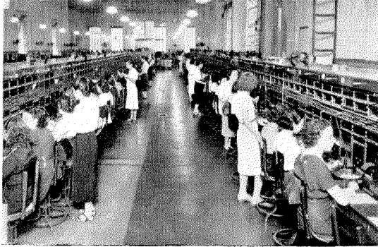
Fig. 4—"Norte" toll sections.
