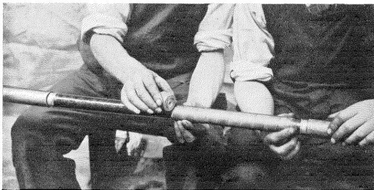
Fig. 2—Lapping on the paper tape.
