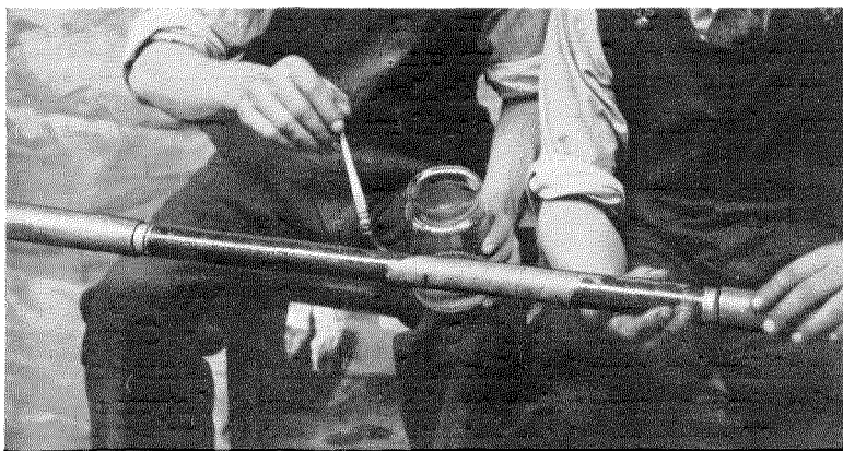
Figs. 2 and 3—Two stages in the fabrication of a styrene joint by the "cold process" using pre-polymerised styrenated paper.
