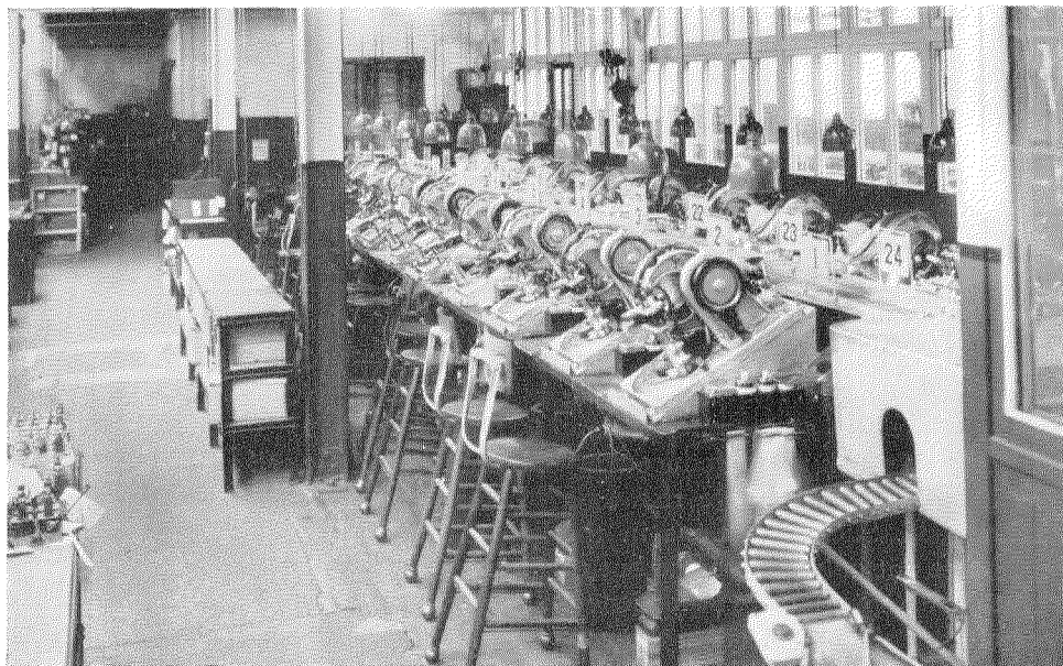
Figure 12—Coil Winding Room.
