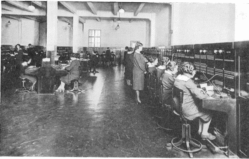
Figure 11— New Toll Switchboards, Barcelona.
