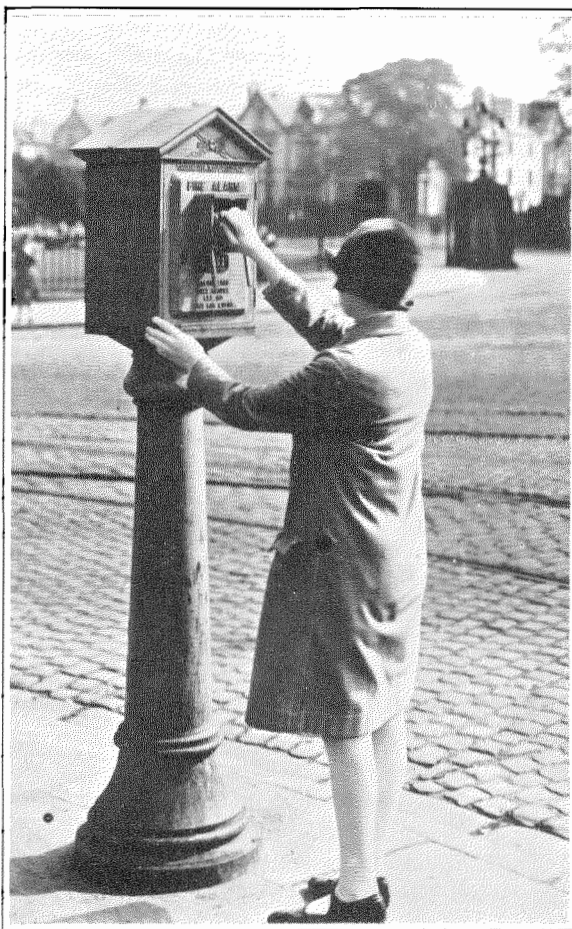
Figure 9—Street Point Apparatus Without Police Signal.
