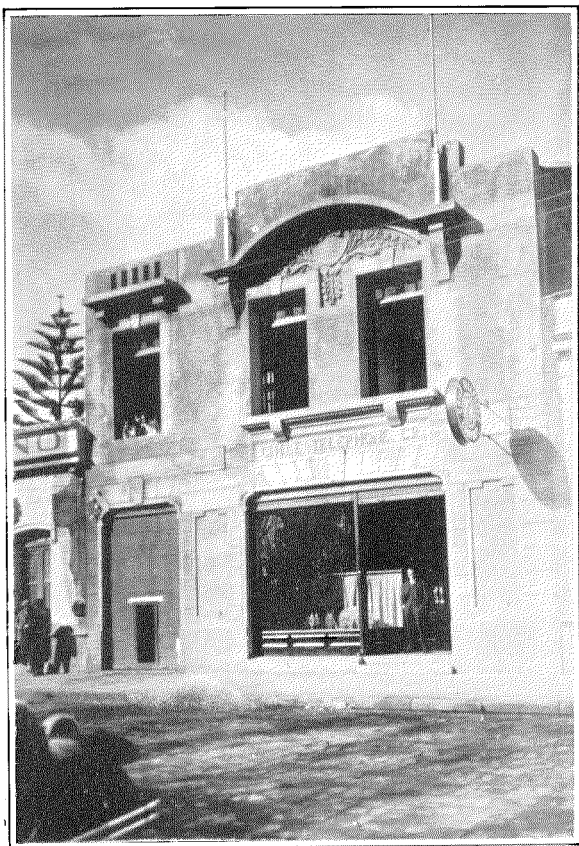
Chillán Central Office Building.
