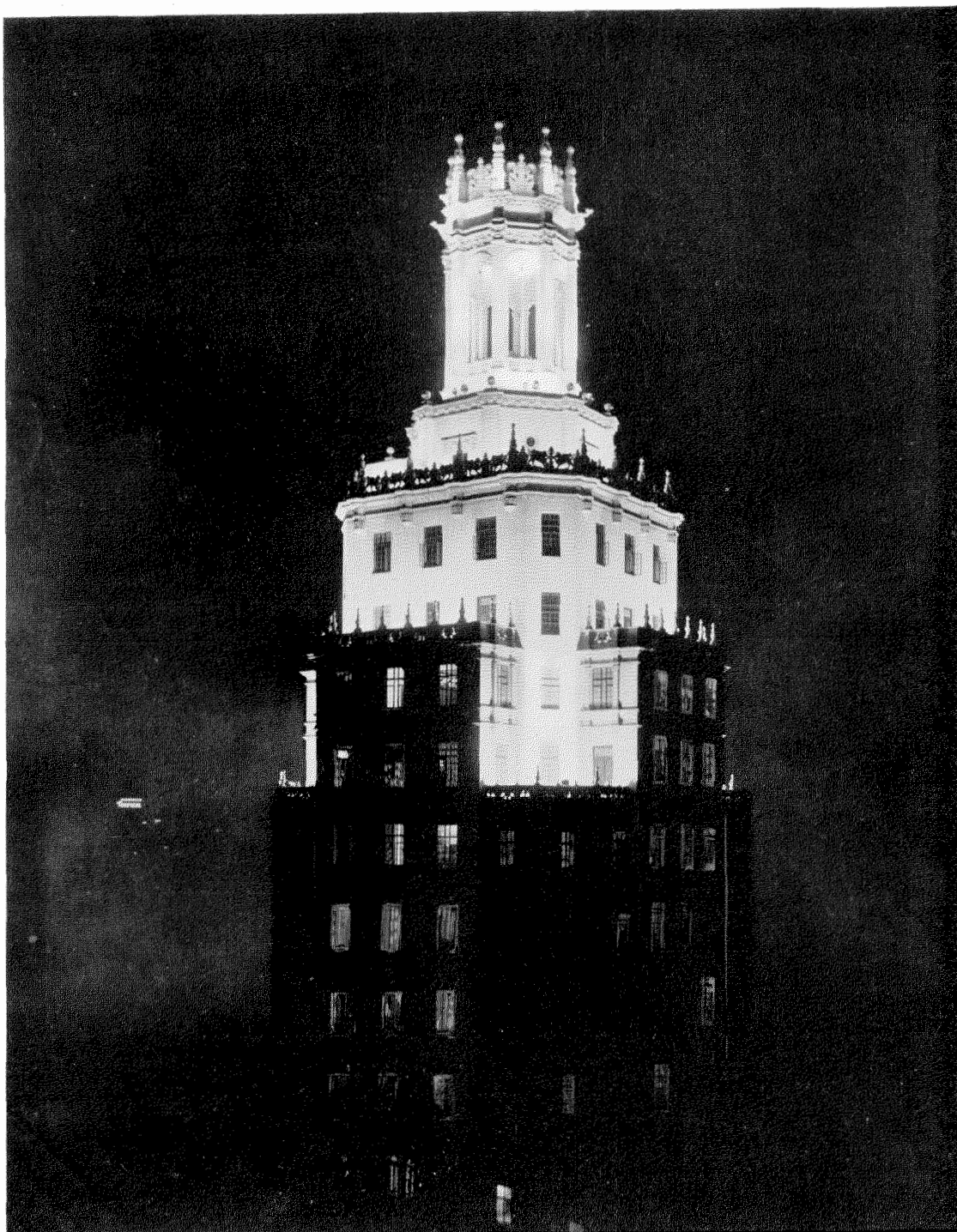
New Building of the Cuban Telephone Company, Havana. It is the highest building in Cuba, consisting of ten stories and a three-story tower. The illustration shows the results of the recent installation of floodlighting equipment.
