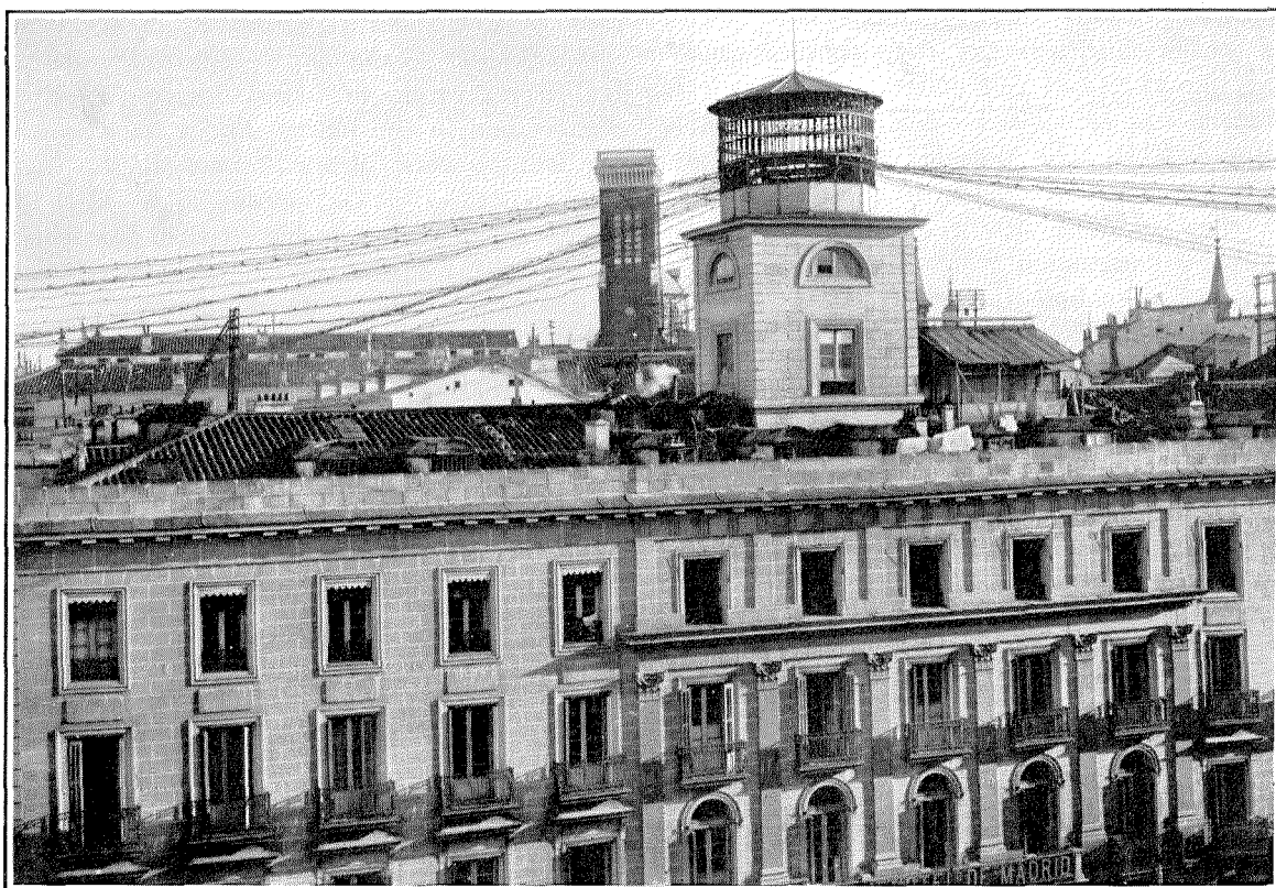
Figure 1—Overhead Wires and Cables Entering the Mayor Manual Exchange, Madrid, through a Tower on the Roof. The housetop construction, typical of the old outside distributing plant, may be seen on the horizon.
