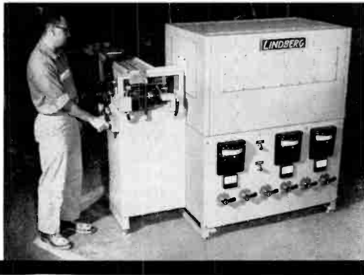
Mechanical Pusher Type Furnace for production of transistors by gas diffusion.
