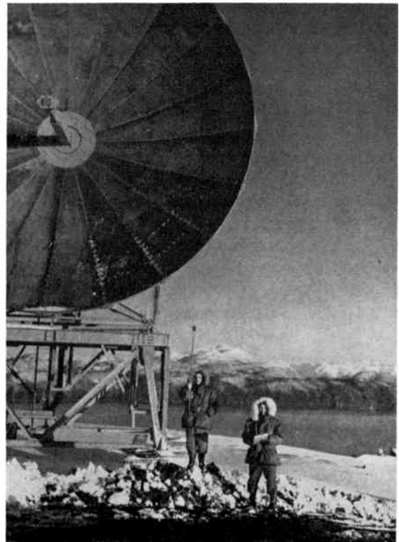
Fig. 5—Tropospheric scatter antennas
