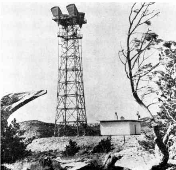
Fig. 3—A TD-2 microwave relay link tower (courtesy of Mountain States Telephone and Telegraph Company).
