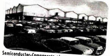
Semiconductor-Components plant . . . world's largest semiconductor manufacturing facility. Construction underway will more than double its size.
