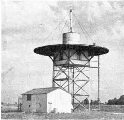
Fig. 2—Omnirange ground facility.
