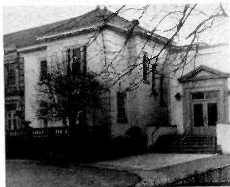
The Conference will be held at the Engineering Societies Building located at McMillan and Woodburn Sts., Cincinnati, Ohio.
