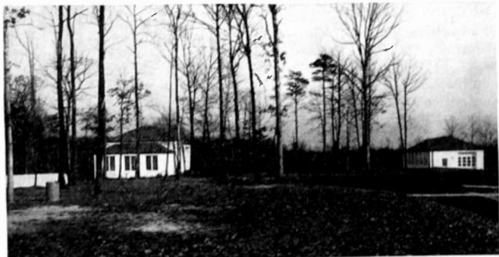
Fig. 7—View looking east, showing the Spherical Field Laboratory, Building 203, and Long Field Laboratory, Building 204.
