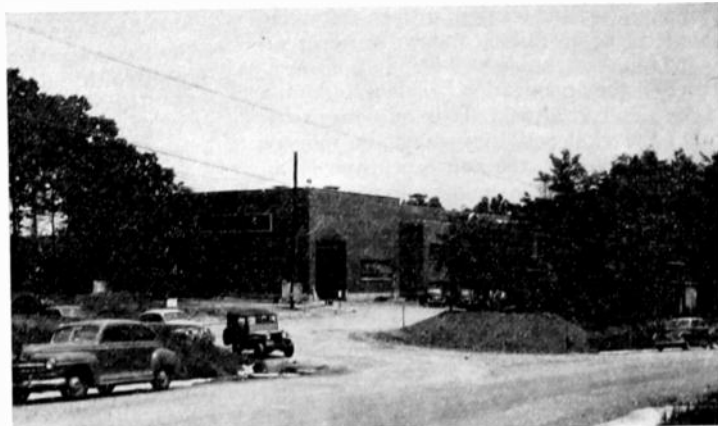
Fig. 9—Supersonic Wind Tunnels Building, view looking northeast.
