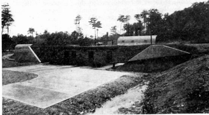
Fig. 8—The Explosives Research Laboratory, one of several located in an isolated area of the Naval Research Laboratory grounds at White Oak, Md., near Silver Spring.
