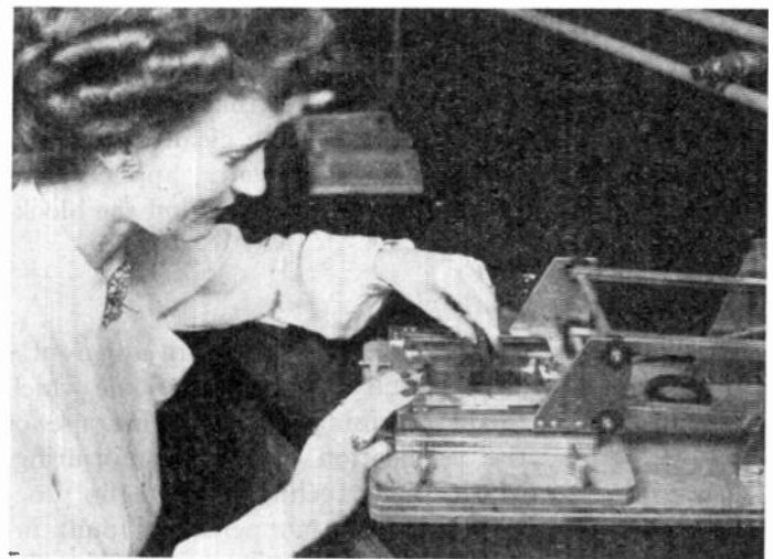
Fig. 12—Application of paint through a stenciled screen. A single smooth stroke of the squeegee is required.
