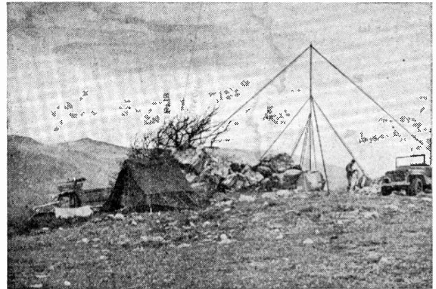
Fig. 12—Transmitter site of radio-relay station in North Africa.
