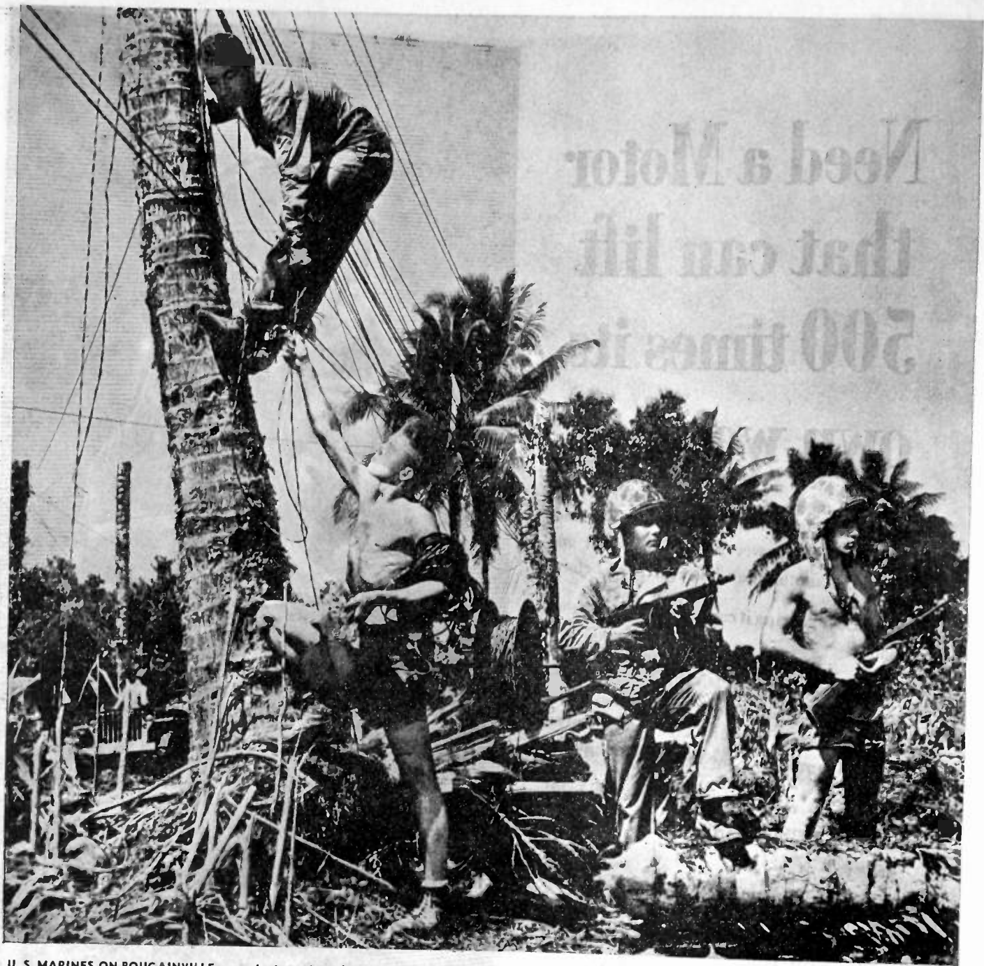
U. S. MARINES ON BOUGAINVILLE use palm trees for telephone poles as they string communication lines. Two stand guard with carbine and sub-machine gun.
