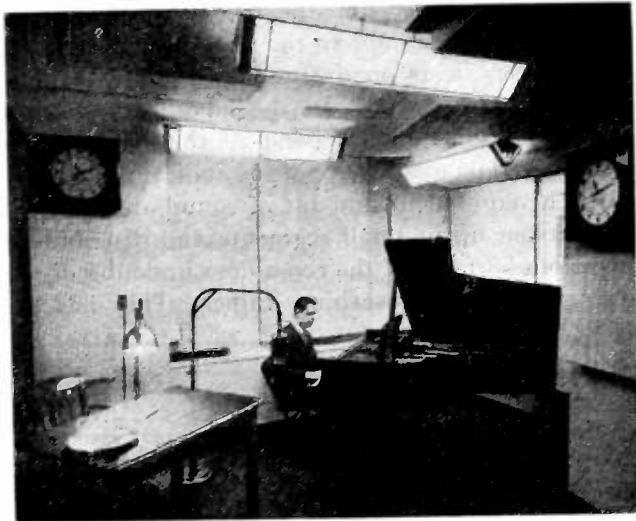
Fig. 4—WOR studio 8 showing sizes and placement of sound-absorbent panels.
