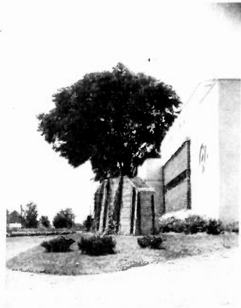
Fig. 4—Sand barricade in front of glass-brick section of CBF transmitter building.
