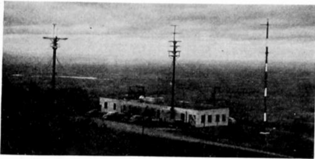
Fig. 1—General Electric frequency-modulation and television transmitter station in the Helderberg Mountains near Schenectady, N. Y.
