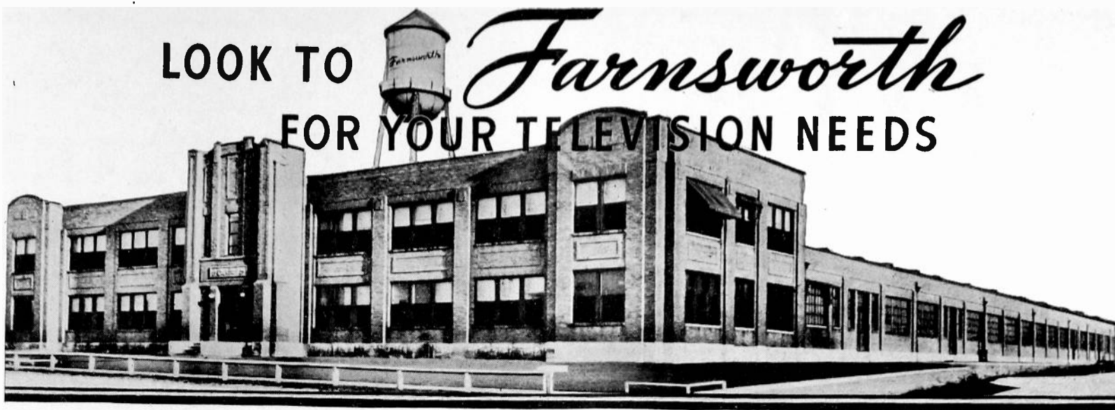
Farnsworth's Fort Wayne plant housing administration offices, research laboratories and special products manufacturing division.
