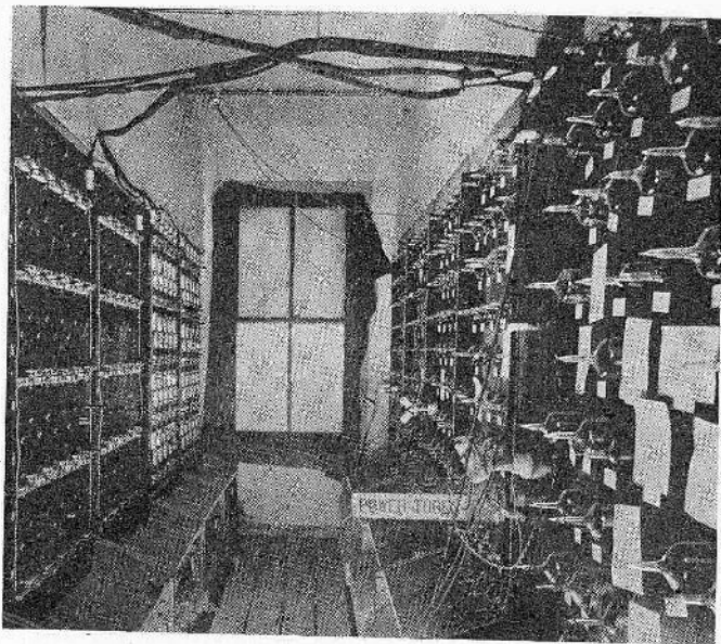
Fig. 2—Power amplifier of the Arlington, Virginia, experimental transmitter, 1915.
