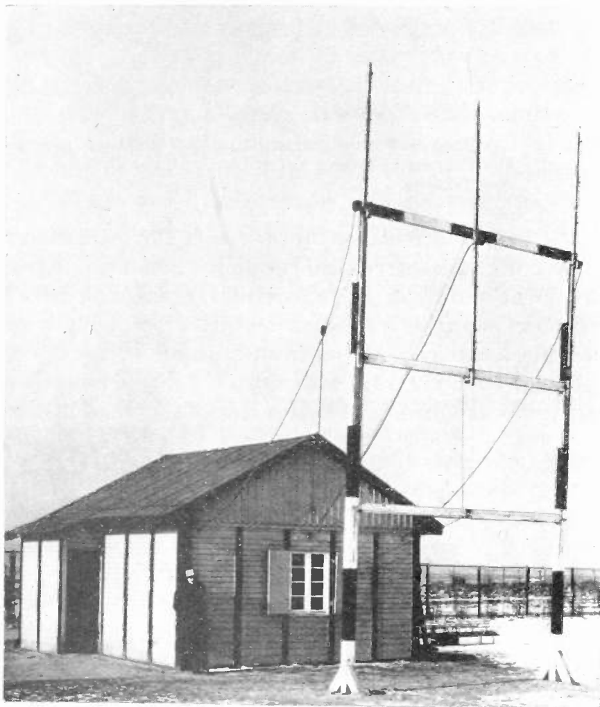
Fig. 3—Ultra-short-wave beacon, Berlin-Tempelhof airport.
