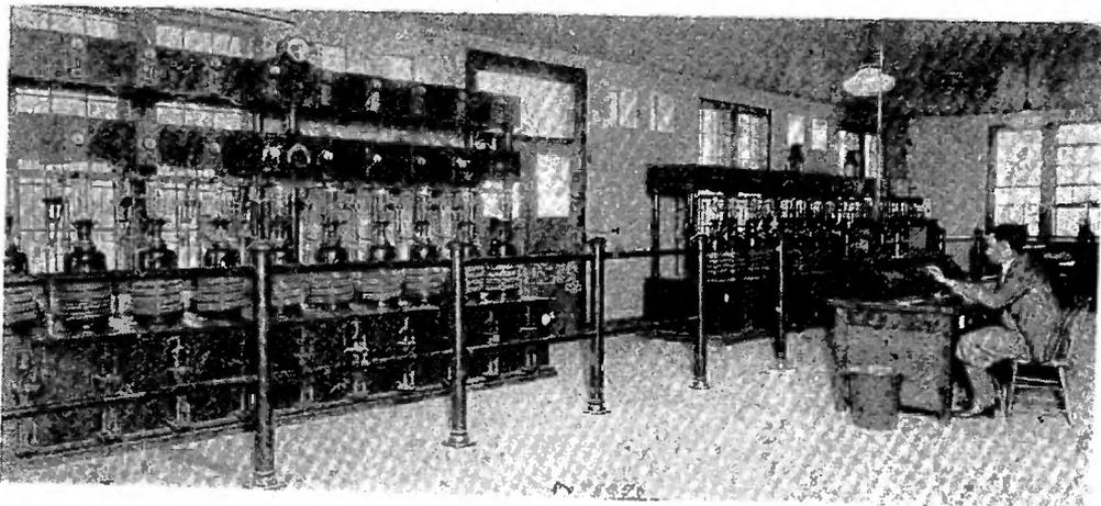
Fig. 29—Broadcast station employing type 50-A transmitter. View shows main transmitter room.
