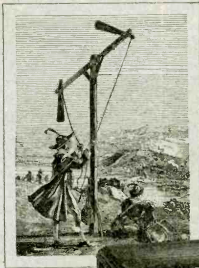
Shortly before the French Revolution Claude Chappe invented a semaphore telegraph system consisting of relays of towers surmounted by movable arms. Messages could be conveyed fifty leagues in fifteen minutes. In August, 1794, the first line was completed between Paris and Lille and on September 1st news of the capture of the town of Condé from the Austrians was transmitted from Lille to Paris.
