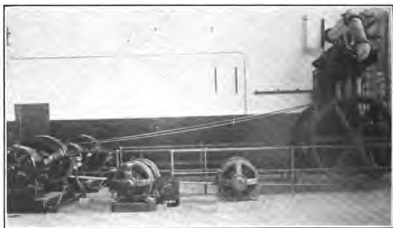
FIGURE 9—Tuckerton Radio Station Dynamo Room.
