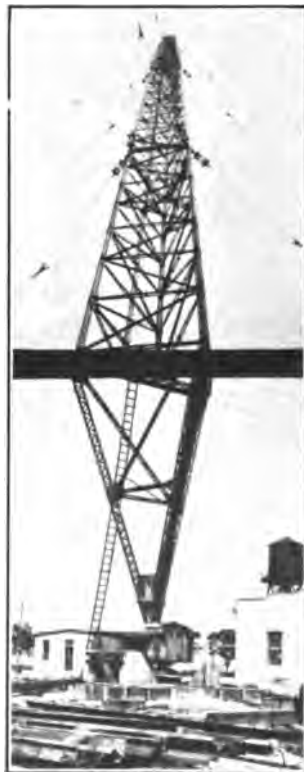
FIGURE 12—View Looking Up Steel Tower.
