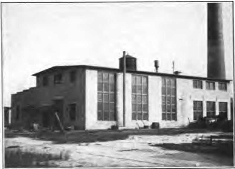
FIGURE 6—Tuckerton Radio Station Power House.
