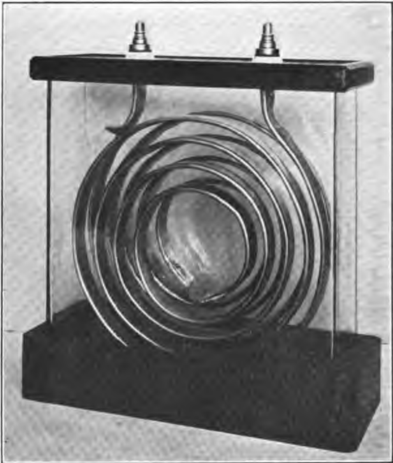
FIGURE 15—Twenty-five Microhenry Inductance Coil Unit, 200 Amperes.
