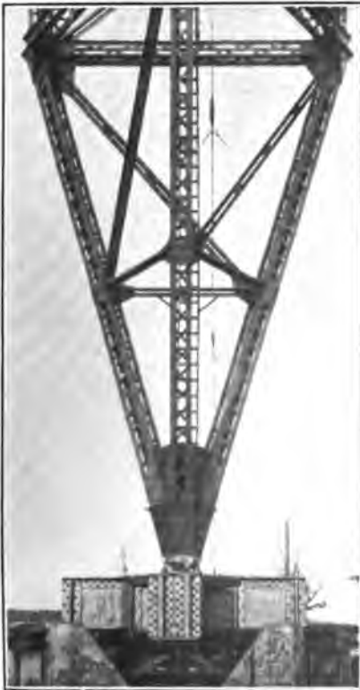
FIGURE 11—Base of Steel Tower Supported on Columns of Glass Insulators.
