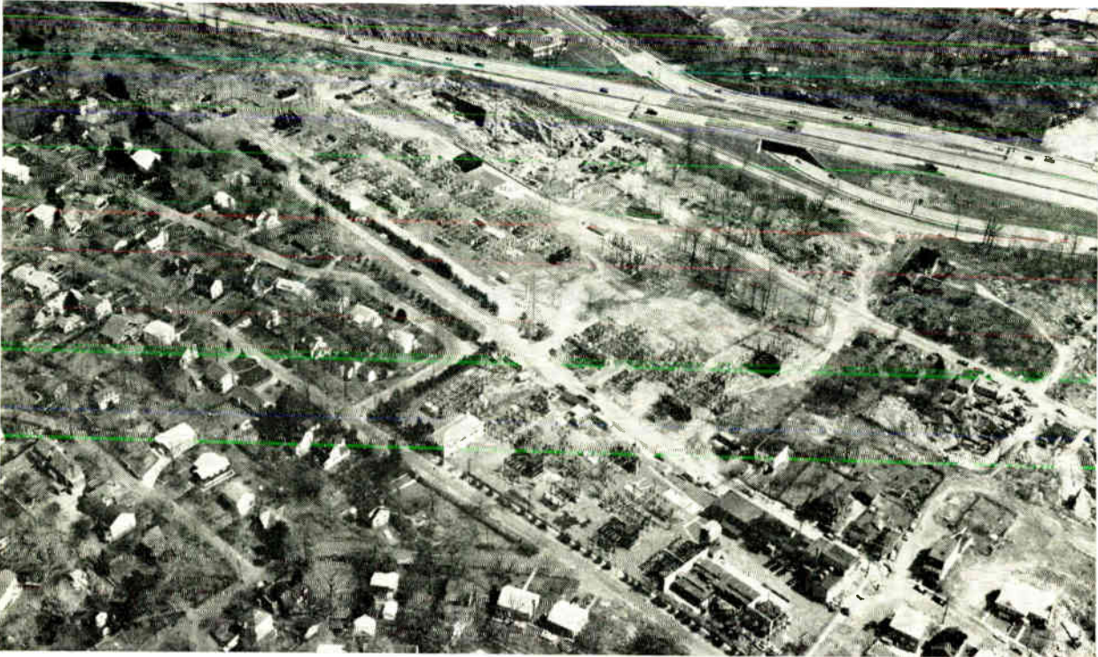
Fig. 26. Sprawling switching station on high rock ledge could make suburban community residents unhappy during and after construction.
