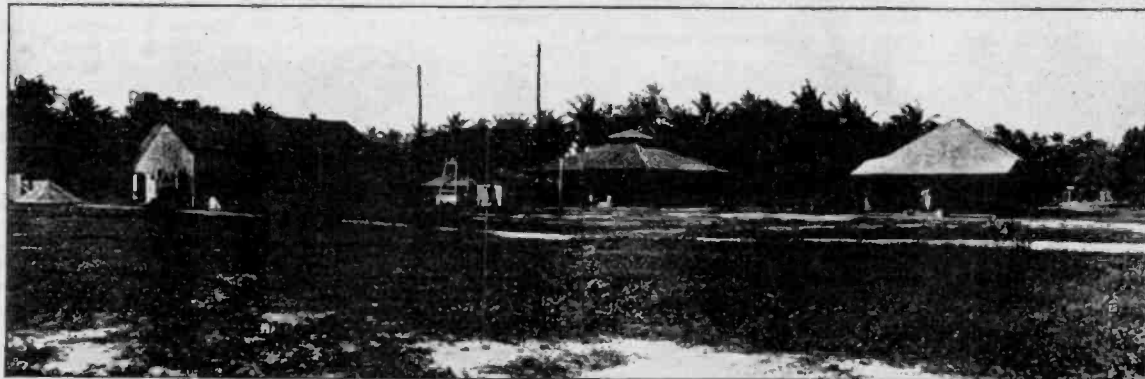
THE RADIO STATION AT SANTA MARTA, COLOMBIA Showing the power house, operating house, and residence for employees
