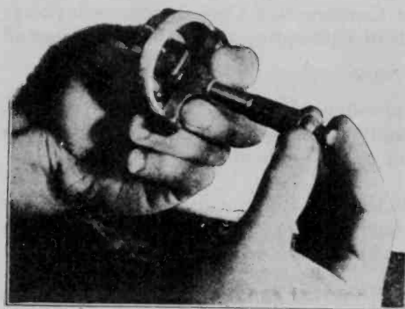
Here We See How the Depth Micrometer Is Used in Measuring Up the Distance of the Pole Faces from the Edge of the Receiver Case.
