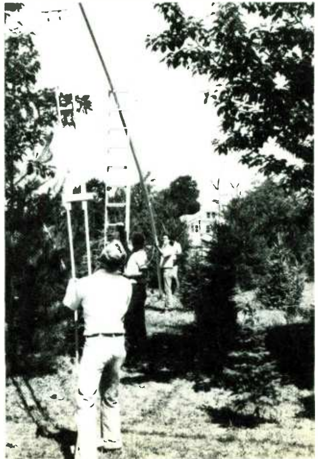
After cutting the antenna back for halfwave operation, we got smart and built a hand held scaffold (foreground).
