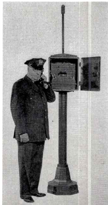
TWO-WAY RADIO CALL BOX AND SELECTIVE SIGNAL LIGHT FOR POLICE AND CIVIL DEFENSE
